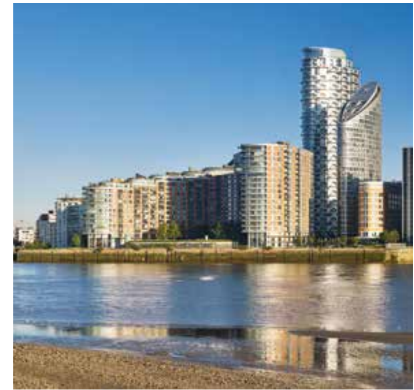
NEW PROVIDENCE WHARF
